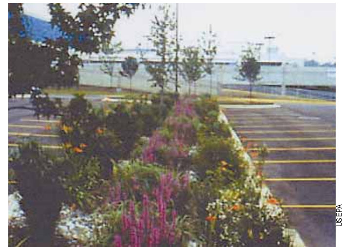
Bioretention landscape in a parking lot in Maryland slows runoff.
